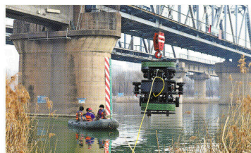
An underwater maintenance robot is lowered to conduct inspection work on a bridge of the Xinxiao-Yanzhou Railway in Jinan, Shandong province, in February. GUO XUELI / XINHUA
